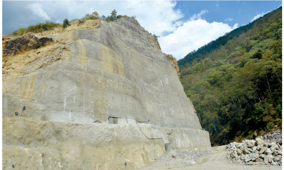
■ A view of the open cut undertaken near the intake site shows complexity of works required to divert water from the Melamchi river
